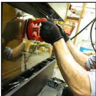
Handle glass with supplied vacuum clamps
